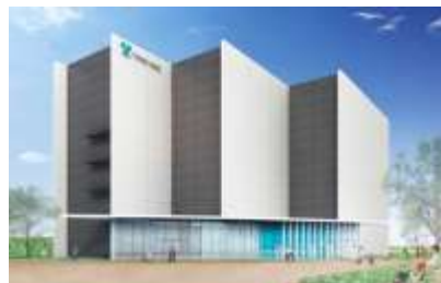
Energy Center, Energy Management System
